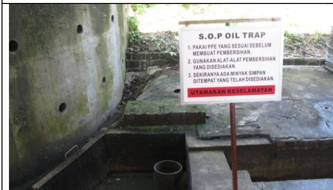
Signages and oil trap at the POM
